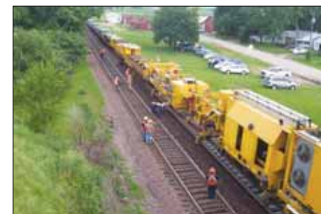
Track Renewal Train (TRT 909)
