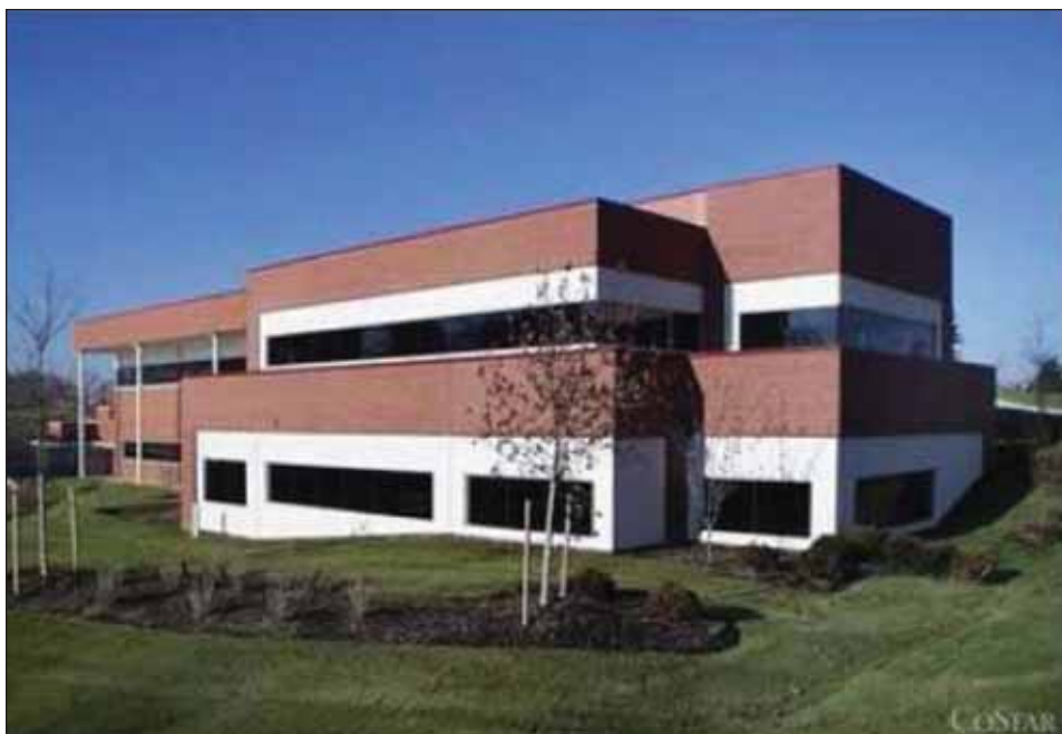
Future home of BMWED, 41475 Gardenbrook Road, Novi, Michigan 48375
