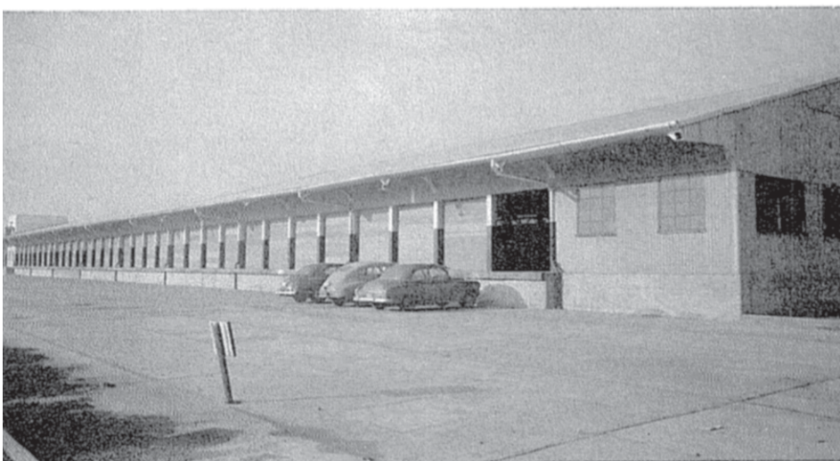
Above: Two view of the million-and-a-half dollar Missouri Pacific freight terminal at St. Louis built by maintenance of way bridge and building forces. This mammoth structure covers more than three city blocks.
