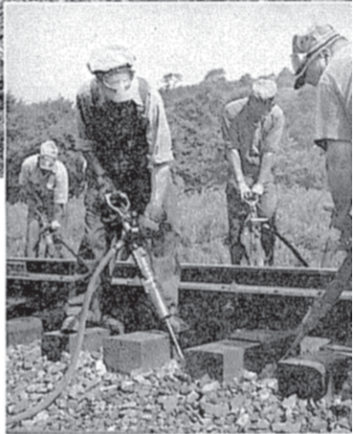
↑ Above: A gang of men surface track with hand tools under the direction of their foreman.
