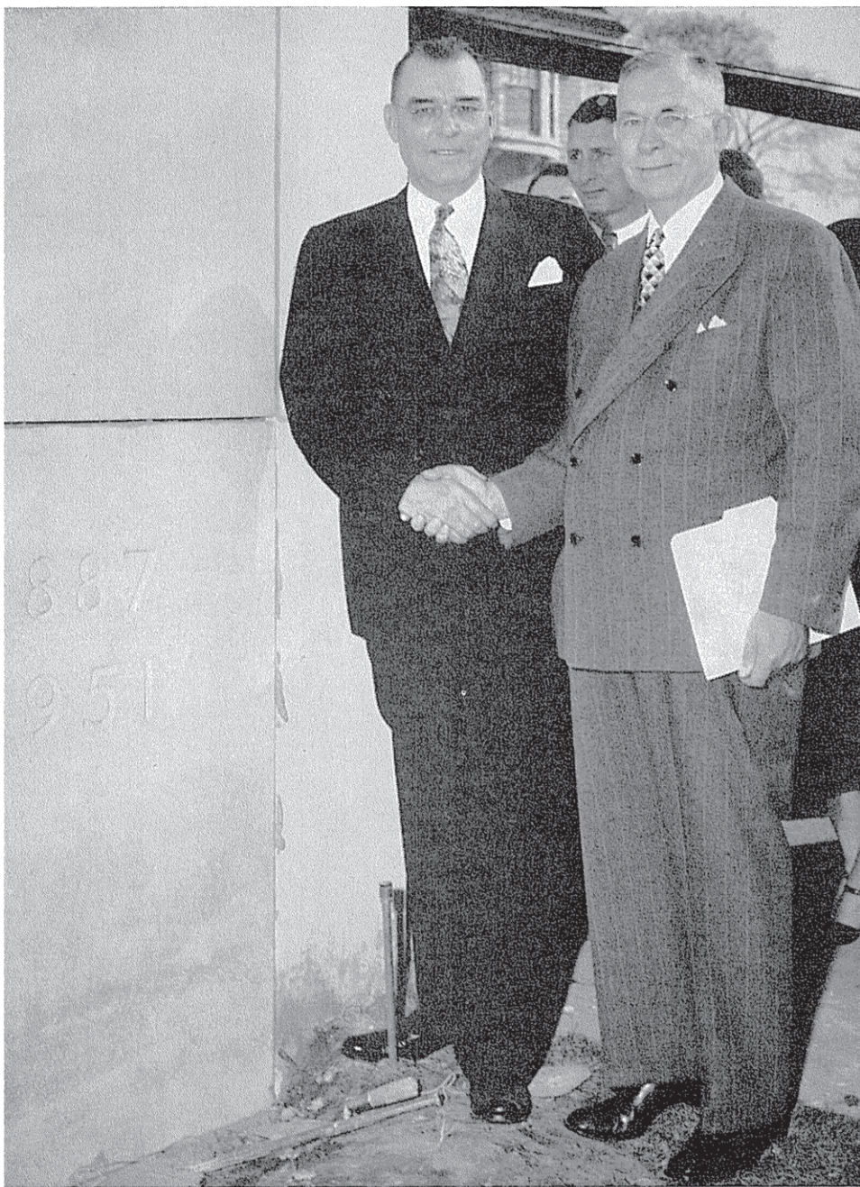
President Carroll and Secretary-Treasurer Shoemake clasp hands after the laying of the cornerstone completes the new headquarters building.
