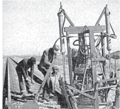
Right: A new development, this one-man four-tool multiple tamper with a track crew packs ballast swiftly and firmly around the ties.
