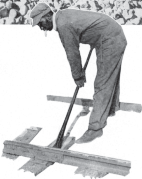
↑ Above: The power-operated spike puller, which removes spikes quickly and easily, has speeded up the maintenance and renewal of America's rail lines.
