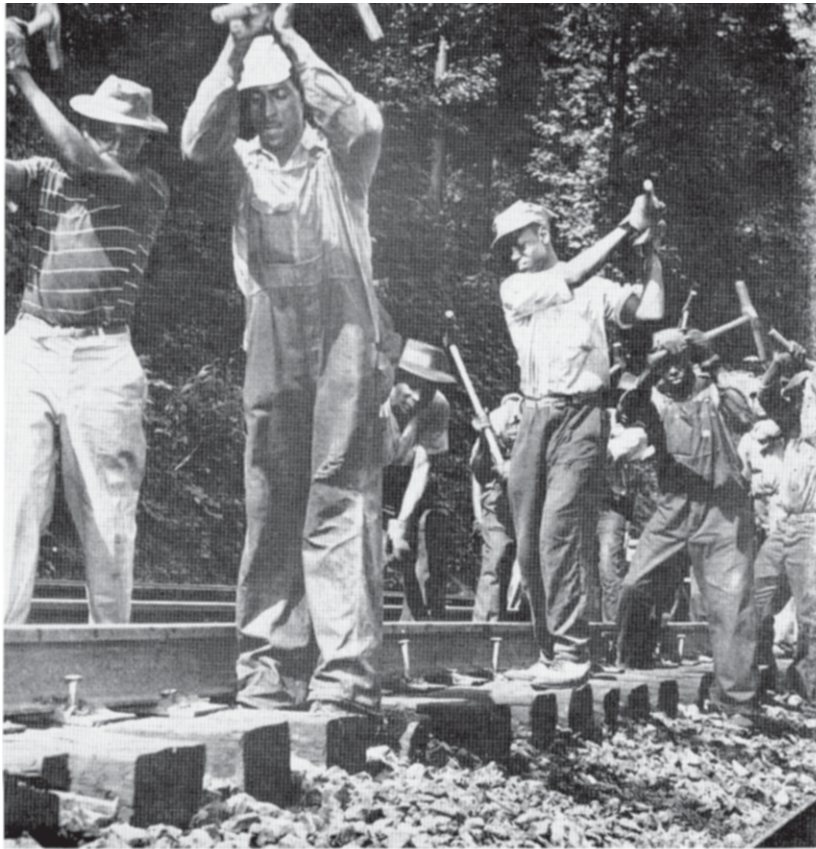
Left: This maintenance crew on the Chesapeake & Ohio at Thayer, West Virginia, drive steel spikes to make the rails secure and safe.
