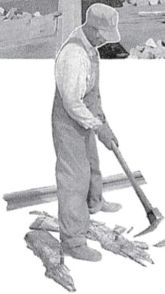
↑ Above: A rail-laying gang at work. After the spike holes have been filled with wooden plugs, ties will be resurfaced by the adzer in the background.
