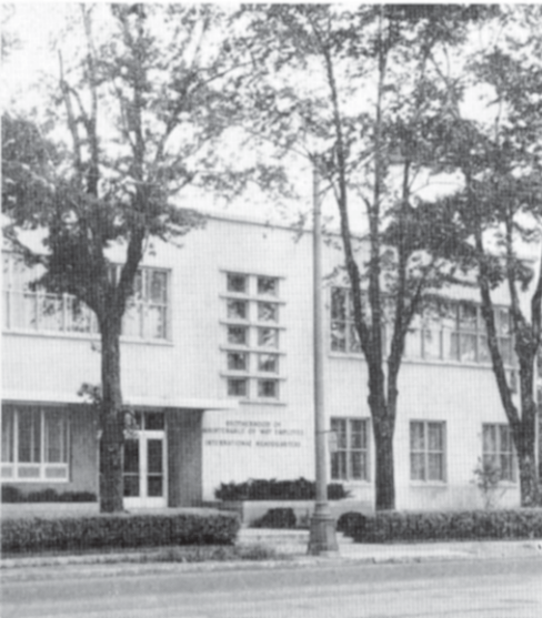
New international headquarters of the Brotherhood at Highland Park, Detroit, Michigan, dedicated October 30, 1951.
