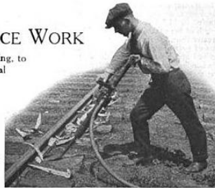
Adzing Ties by Compressed Air
